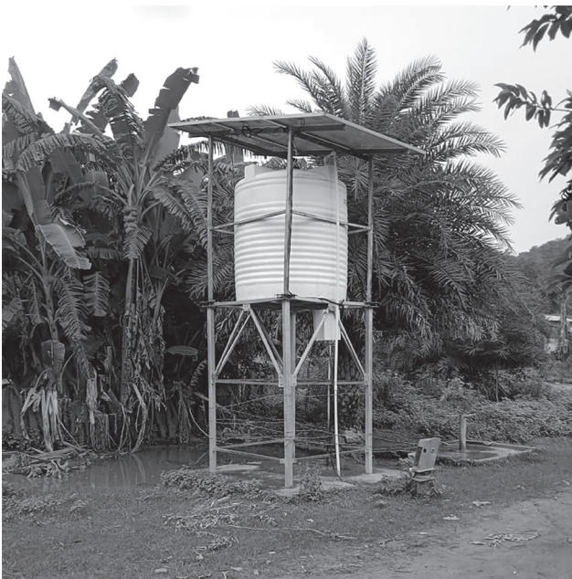
In frame: Solar water tank installed
