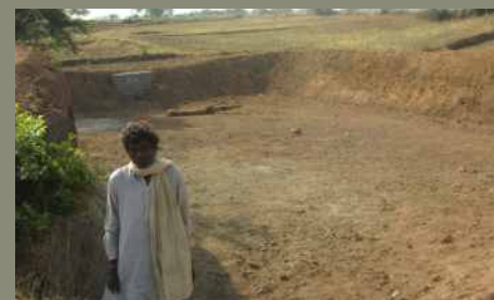
The farm pond nearing completion in Chipani village.
