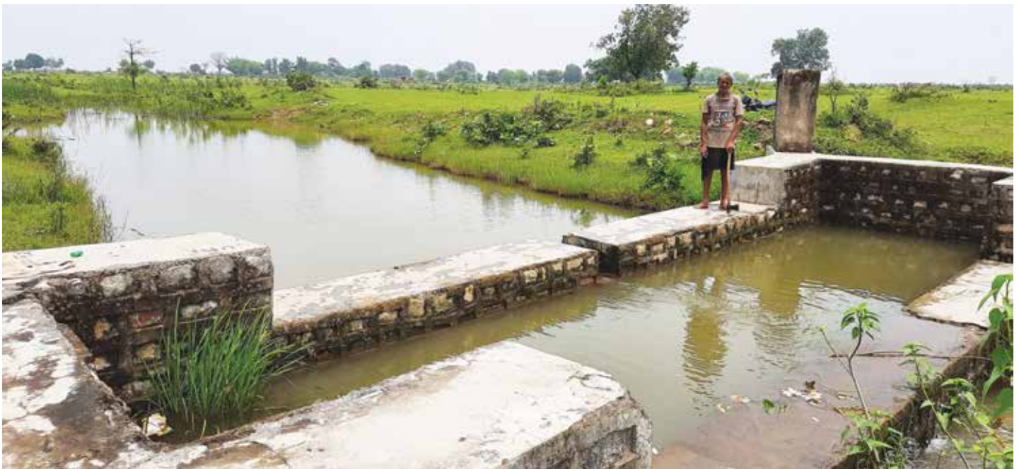
A check dam constructed in Chitrakoot, Uttar Pradesh
