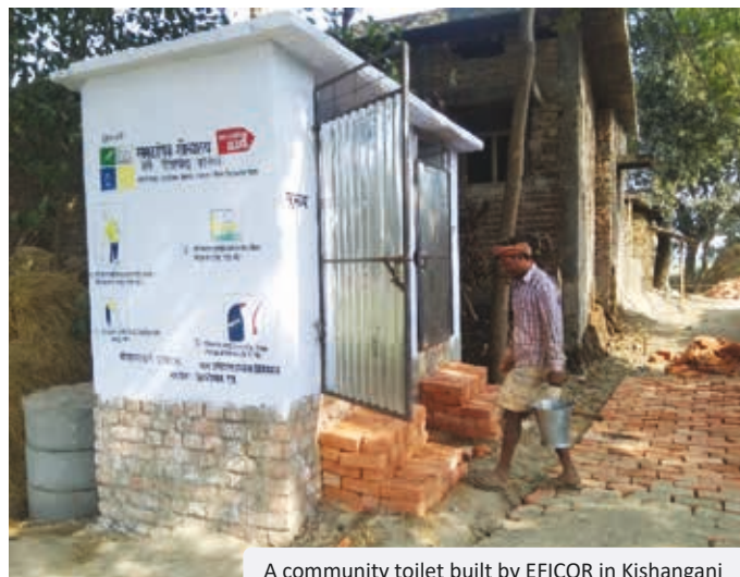
A community toilet built by EFICOR in Kishanganj
