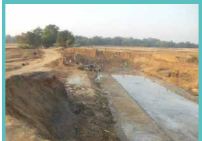
The bridge at Tonda Janboguda village under construction
